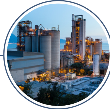
Chemical Process Plant
